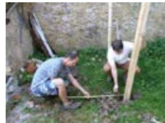
3) Fix the pillars in the way that the bigger ones stay in one side (left or right). Use rocks to fix them until the job is finished.
