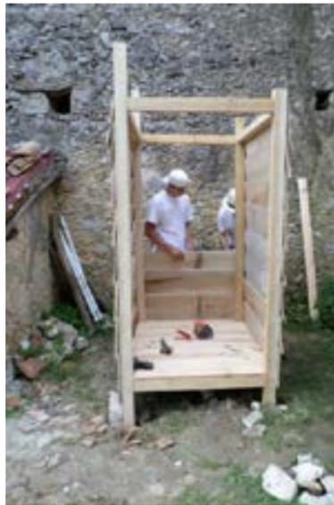
9) Now you will fix the planks to build the walls. Fix the first one from the bottom. The second plank must be fixed 3 cm overlaid from the first one. Repeat the process to build the other walls.
